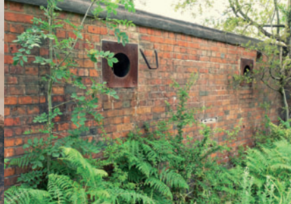
Pillbox at Bouldnor Battery
